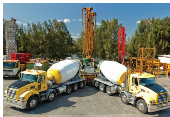
Figure 10.1 – Truck Mounted Transit Mixers delivering Concrete to a Pump on Site
