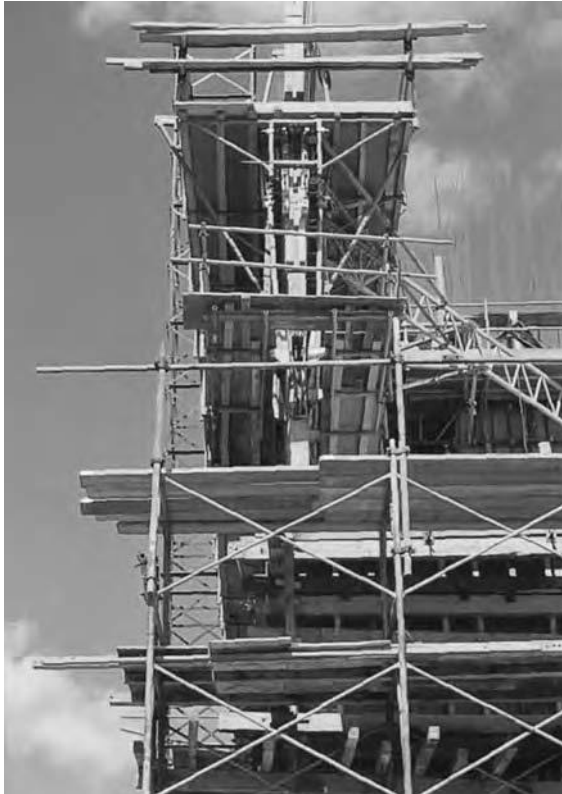
Figure 27.9 – Slip-forming a Vertical Element
