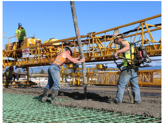
Figure 12.17 – Immersion Vibrator in Use on Slab 12.8
