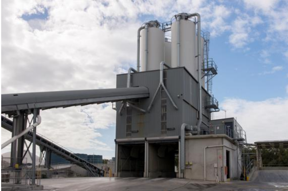
Figure 9.1 – Typical Modern Concrete Batching Plant
