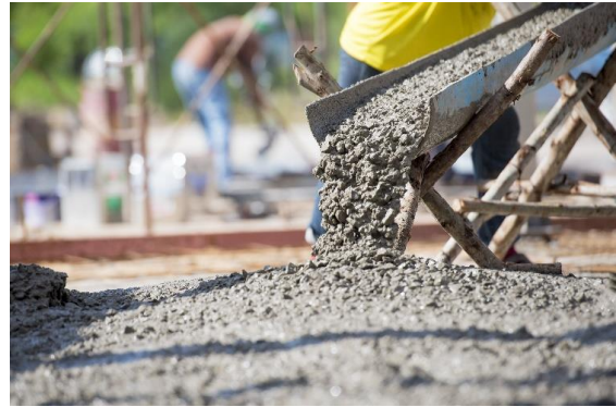
Figure 12.3 – Delivery from a Transit mixer Chute is the Quickest, Most Convenient and Economical Method of Distribution
