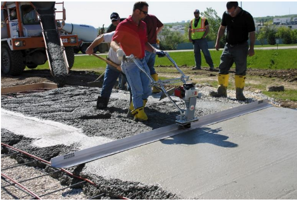
Figure 12.18 – Vibrating Screed in Use 12.9
