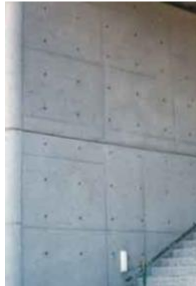
Figure 16.8 – An Even Tie bolt-hole Arrangement will enhance the Overall Surface Appearance
