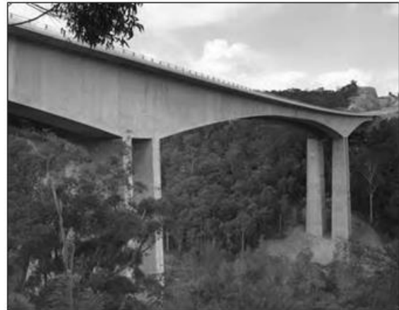
Figure 11.7 – Multi-strand, Post-tensioned bridge, Mooney Mooney, NSW
