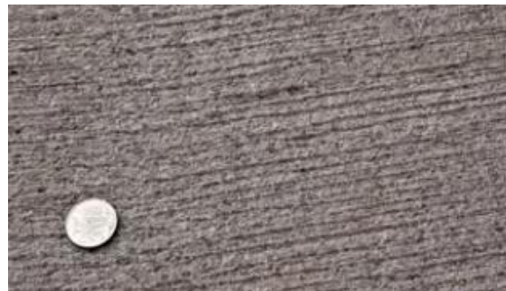
Figure 14.7 – Broom Finishing helps to provide Skid Resistance
