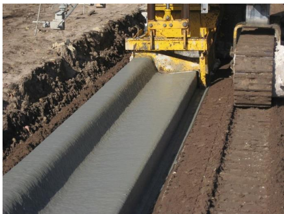
Figure 19.8 – Kerb Construction 19.3
