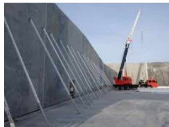
Figure 20.23 – Bracing Panel while Construction Progresses
