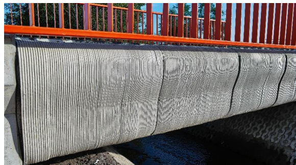
Figure 24.9 – 3-D Printed Bridge, Extrusion-based Technique 24.9
