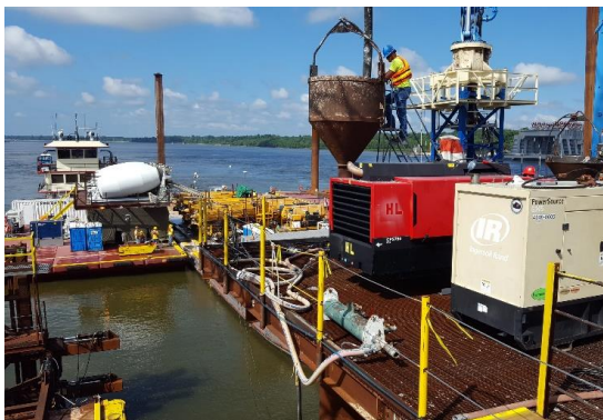
Figure 12.9 – Tremie Pipe being filled from Above-ground Hopper 12.4
