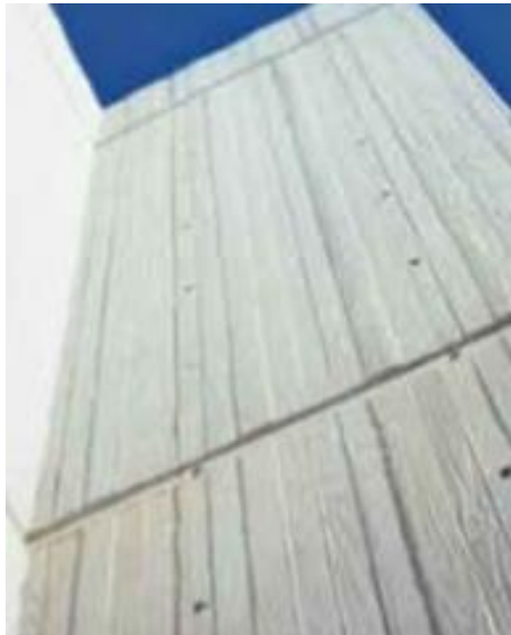
Figure 16.3 – Example of Carefully detailed Off-form Concrete
