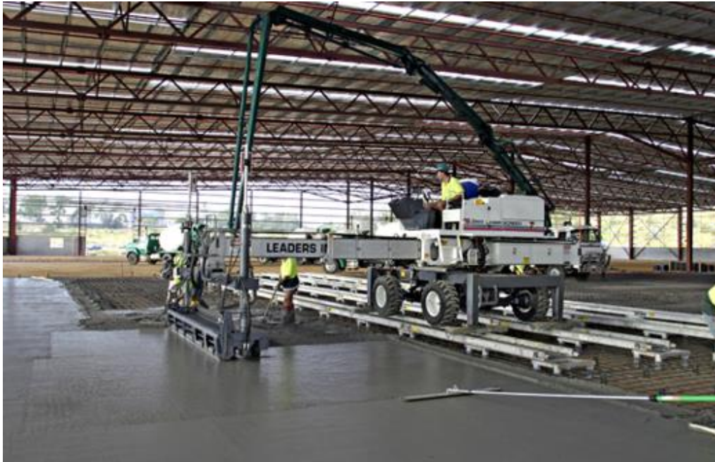
Figure 14.2 – Typical Machine-mounted Beam Screed
