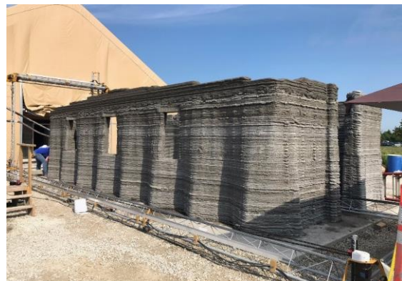
Figure 24.8 – 3-D Printed House, Extrusion-based Technique 24.8
