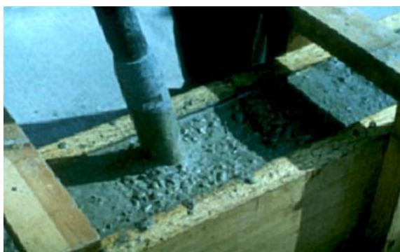
Figure 13.3 – Using an Immersion Vibrator
