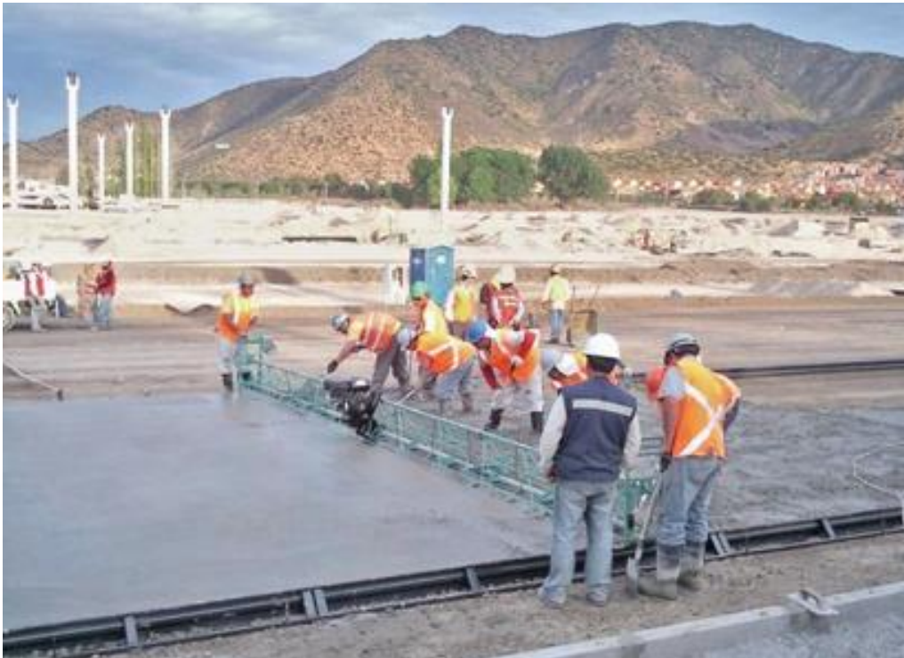
Figure 14.1 – Typical Trussed Vibrating Beam Screed
