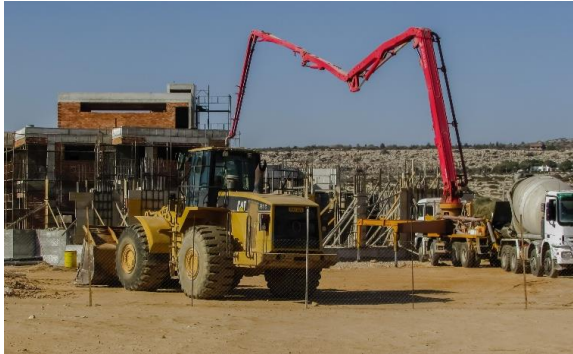
Figure 12.2 – Access to the Site (and particularly the ease with which delivery vehicles can move on and off it) has a Significant Influence on the Overall Concrete Supply Rate 12.1
